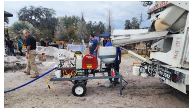
Cretefoamer Model LV-3 on the job. Portland cement and water slurry provided by two cubic yard “short load” ready-mix truck.
